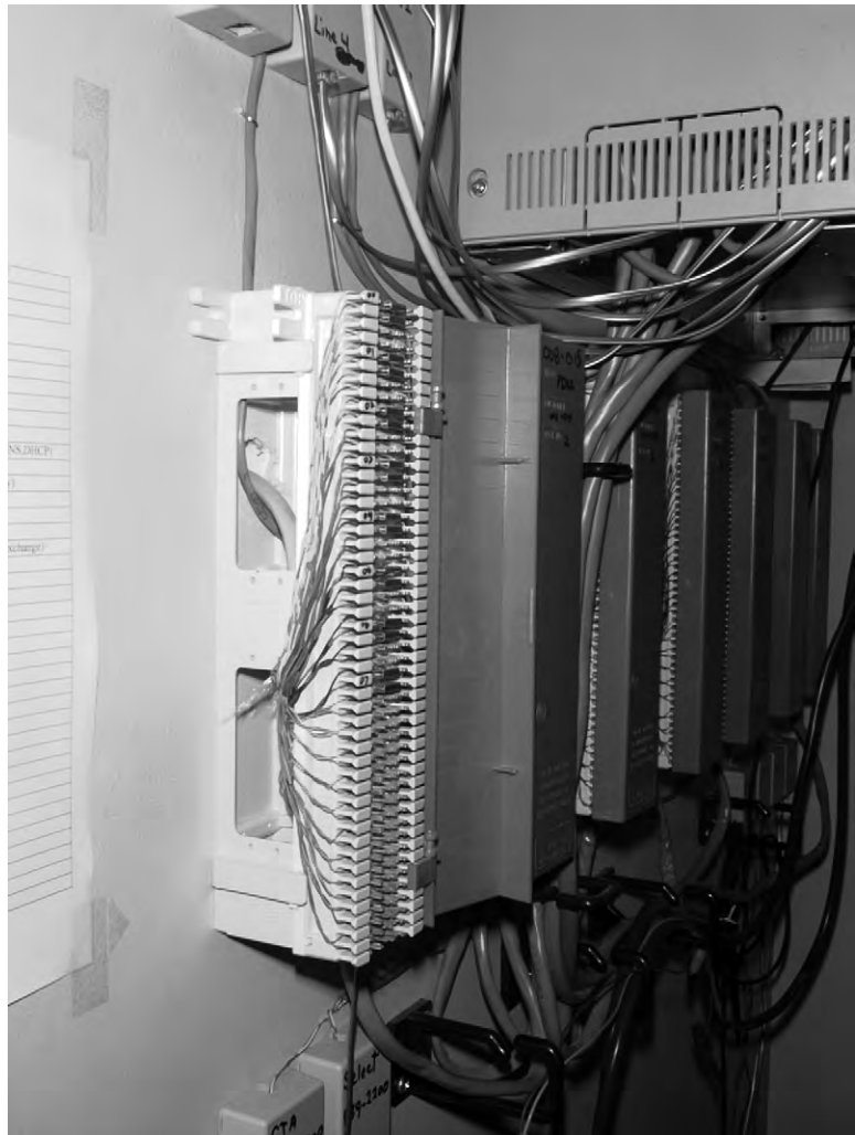
FIGURE 7.21 A 66-block used for voice applications
