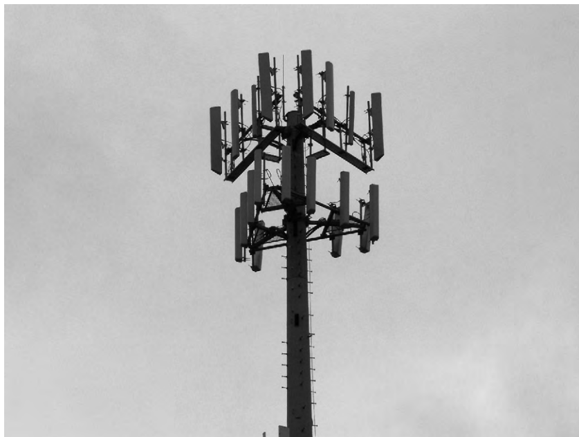
FIGURE 30.15 Antennas on a cell tower
